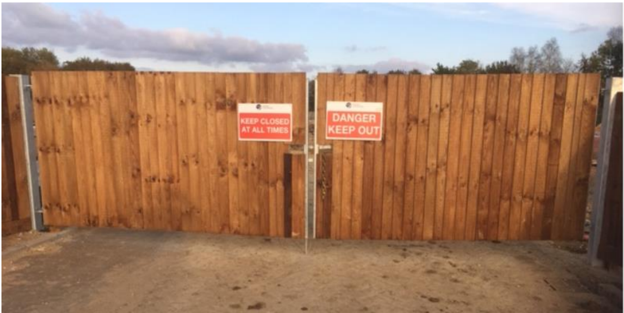
Figure 15 – typical construction compound fencing
